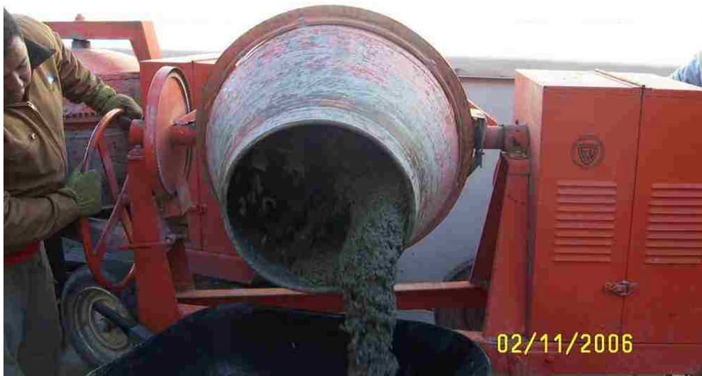
Figure 3.2. Mixing of fresh concrete
